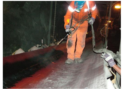
Application of Rhino Tuff Stuff (note overlap)
