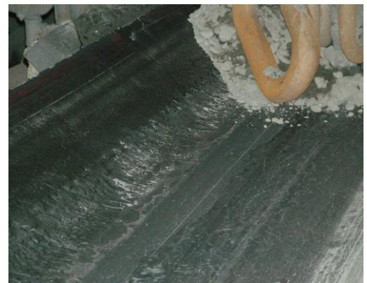
After repair and in operation
