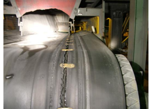
Before repair and with staples fitted
