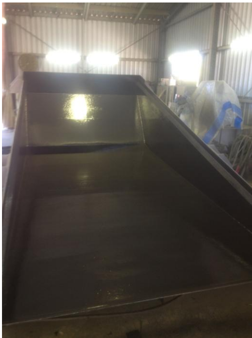
Completed deslime underpan, spray applied with RhinoGuard 2195
