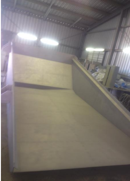
Deslime underpan preped and primed with RL315
